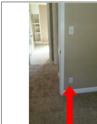
No power present at outlet
