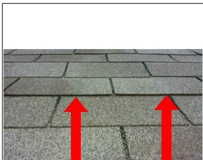
Loose tab attachment in various areas, recommend qualified contractor evaluate
