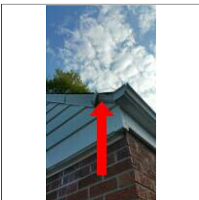
Recommend repair of loose aluminum trim west elevation
