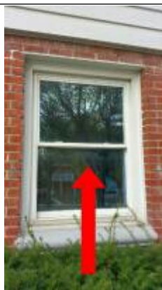
No screen present east elevation
