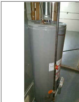
Heavily corroded and not lighting recommend evaluation.
