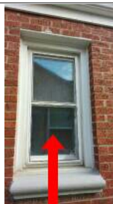
Recommend repair of torn screen south elevation
