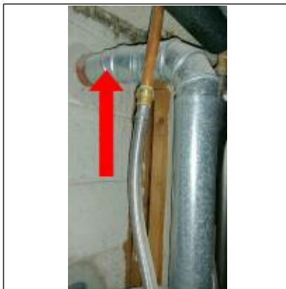
Recommend lining of chimney, hot water heater only appliance vented into clay flue
